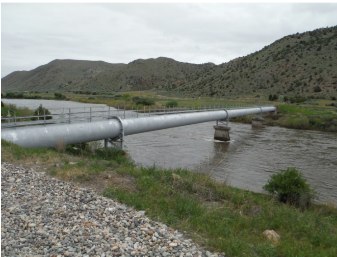
Siphon over the Missouri River on East Canal
