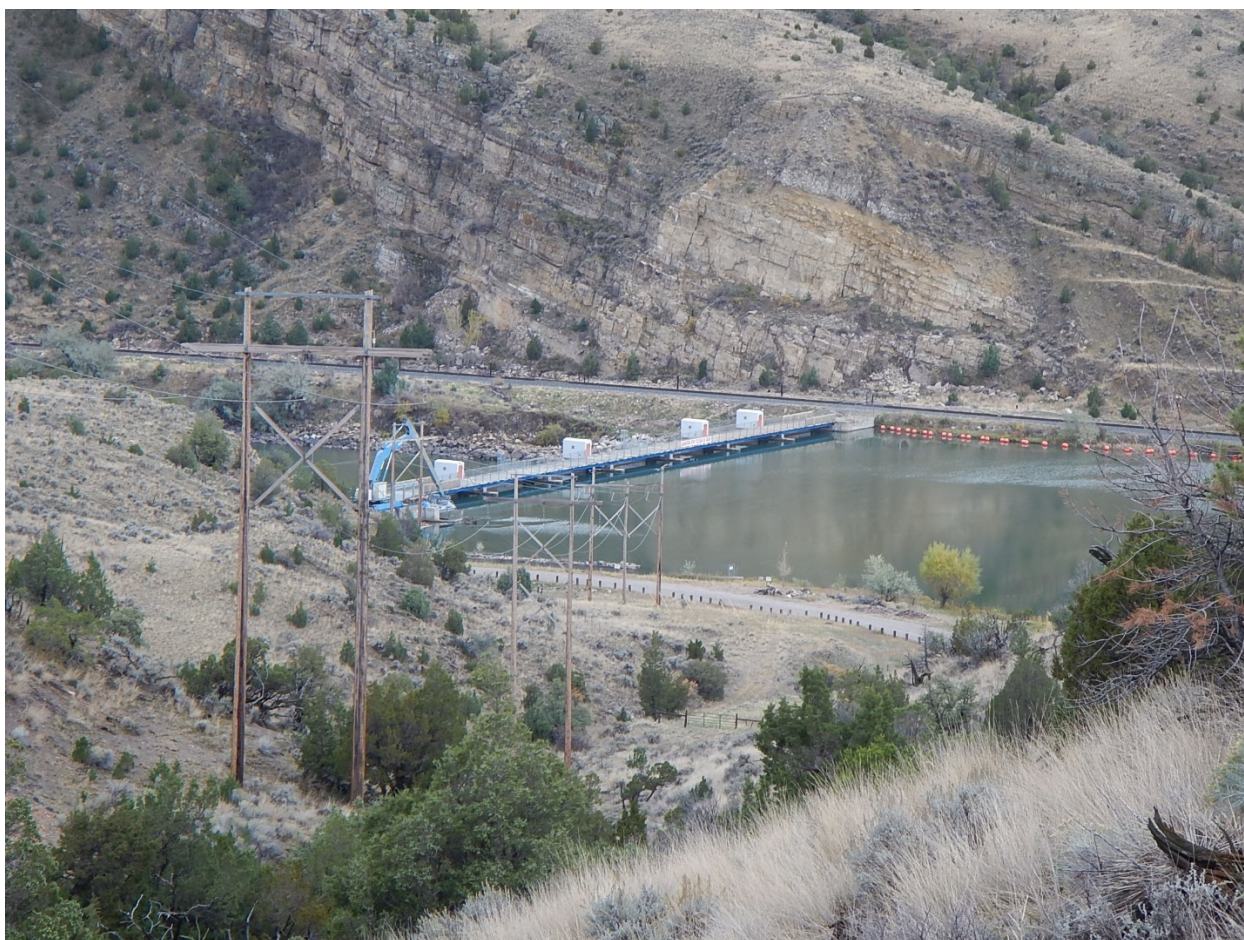
Broadwater Power Project, Missouri River near Toston, MT
