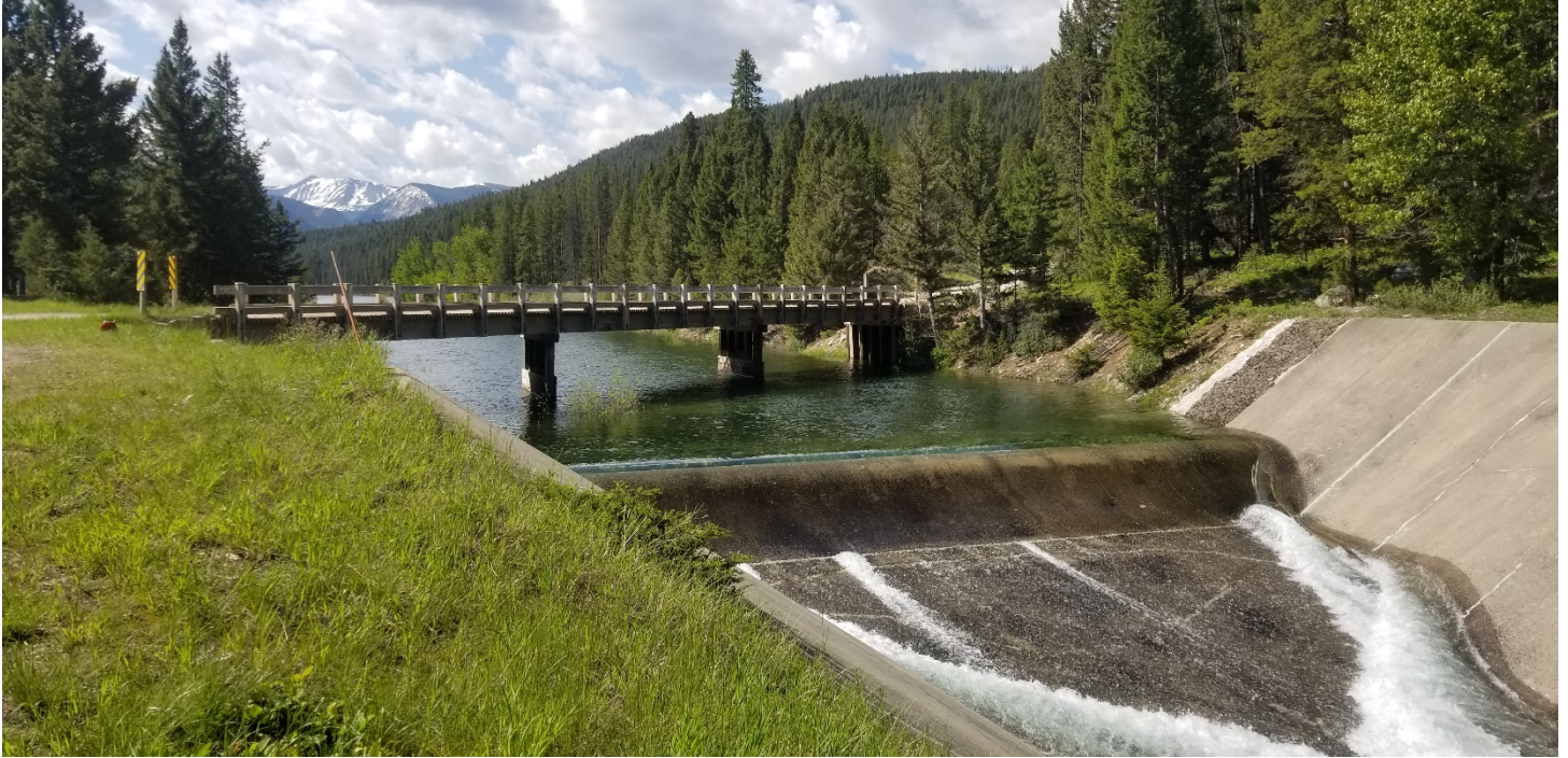
East Fork of Rock Creek Dam Spillway
