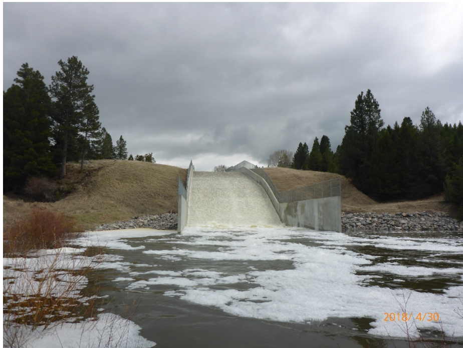
Nevada Creek Dam Spillway (Powell County)
