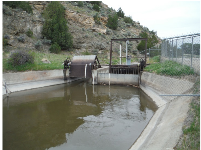
Gates at main canal end, splits into East-West Canals
