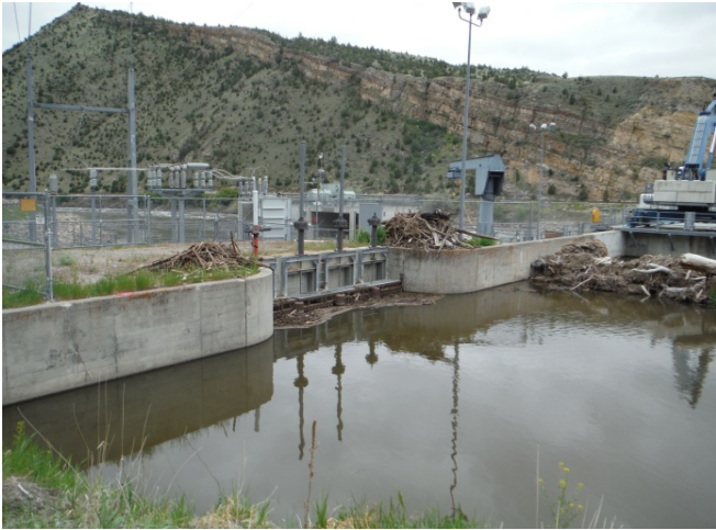
Canal head gates at diversion point (Toston Dam)
