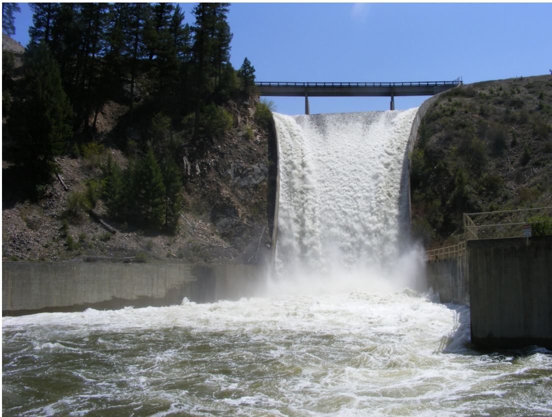
Painted Rocks Dam Spillway
