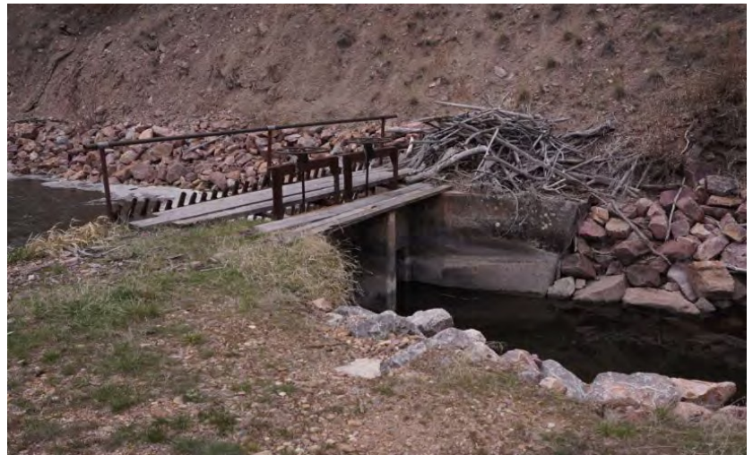
Existing Allendale Canal Intake on Flint Creek
