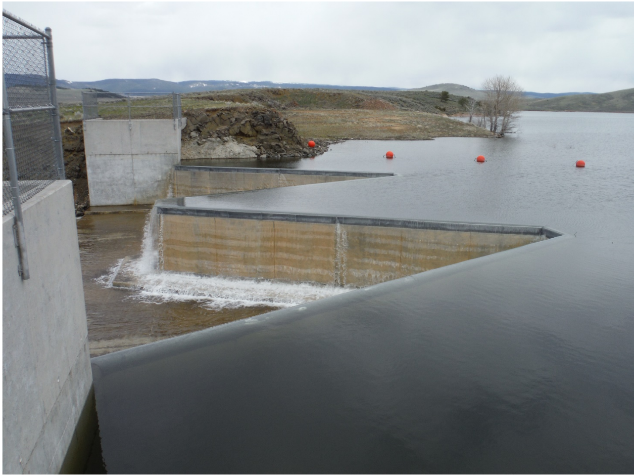
North Fork Smith River Dam, Meagher County
